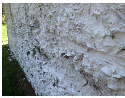
Tabby is made by burning oyster shells to create lime, then mixing it with water, sand, ash and broken oyster shells.
